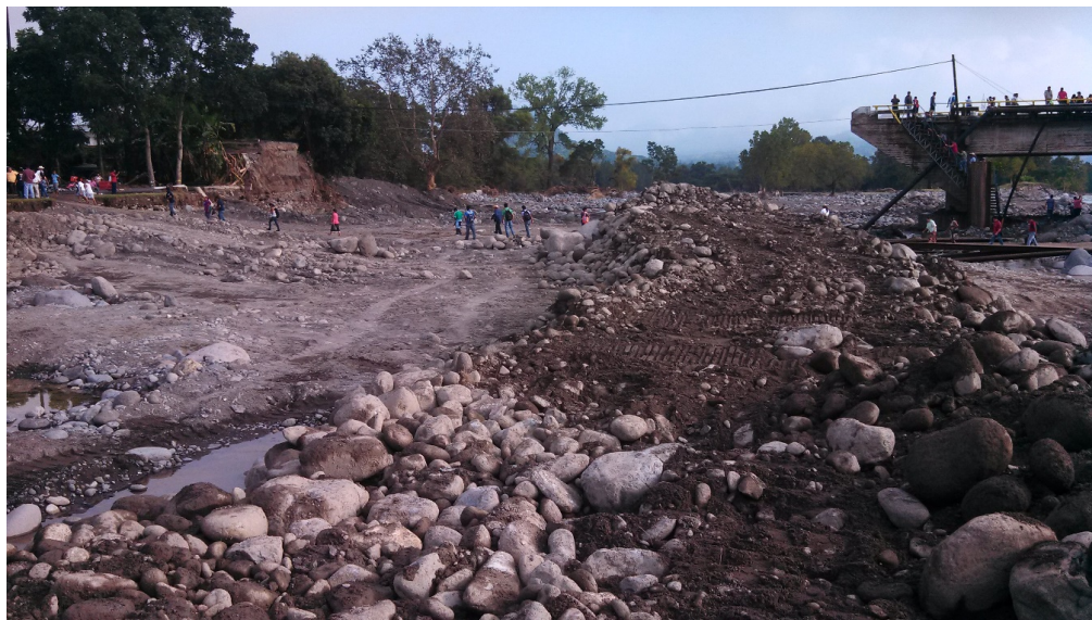
Figure 7. Consequences of fast-flowing rivers during the flood season, causing the rupture of a bridge in the Misantla River, generating social isolation among neighboring populations.
