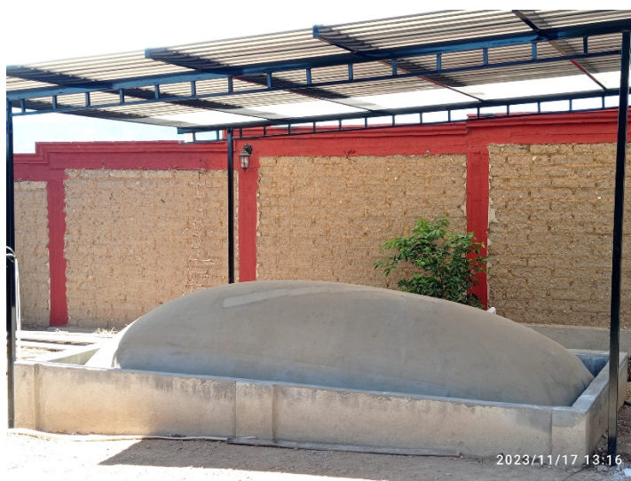
Figure 1. A tubular or bag-type biodigester with a liquid volume of 10 m 3 was used in the present study
