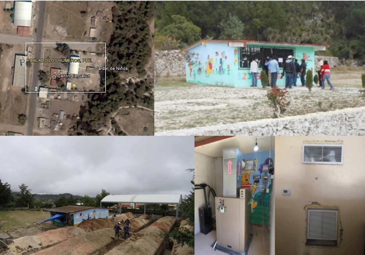
Figura 7. SBCG para Kinder, bomba vertical, GeoComfort
